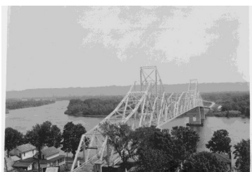
IA-9 border bridge at Lansing, IA. Black Hawk Bridge
