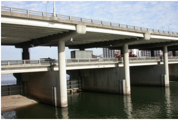
5 in 1 Bridge on I-380
